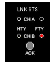
Channel - B Link Status is Faulty
