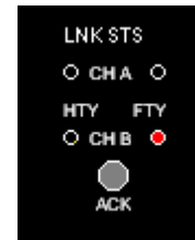
Channel – B Link Status is Faulty
