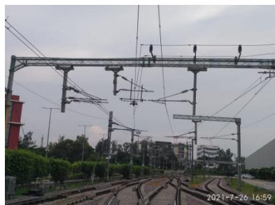
HDPE NET ON PORTAL
