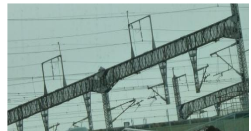
JAPAN RAILWAY-NYLON NET ON PORTAL BOOM & DROP ARM
