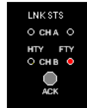
Channel – B Link Status is Faulty
