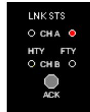
Channel – A Link Status is Faulty
