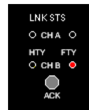
Channel - B Link Status is Faulty
