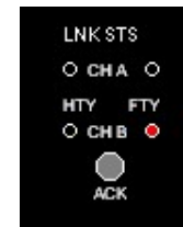
Channel - B Link Status is Faulty
