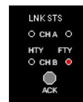
Channel - B Link Status is Faulty
