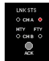
Channel - A Link Status is Faulty
