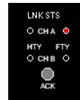
Channel - A Link Status is Faulty
