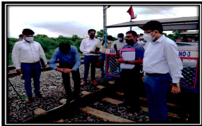
CRS inspection in BLSN_ANMD Section.
