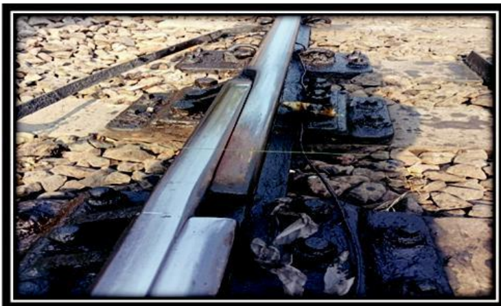
Gap Measurement of SEJ
