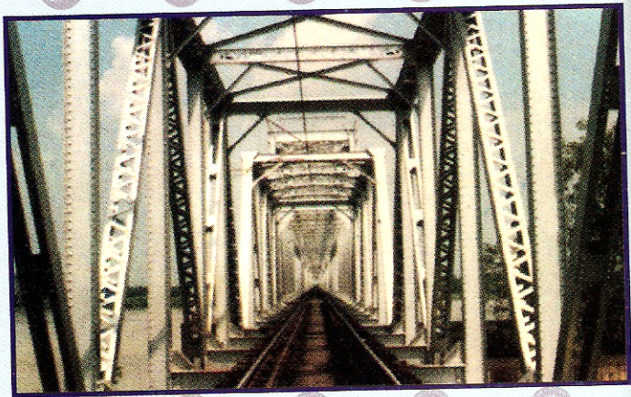
Track on Bridge and in Tunnel on S.E. Railway
